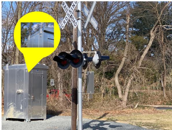
Since 2009, the Signal Department has assigned its supervisors yearly initiative projects to install power indicator lights at grade crossings equipped with automatic warning devices. These crossings all receive commercial power much like we all have at our homes. We use this commercial power to charge batteries; these batteries power all of the warning devices at the crossings.
