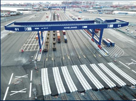
On January 7, 2019, the Port Authority of New York & New Jersey opened the new Global Container Terminal on the site of Conrail's Greenville Yard in Bayonne, New Jersey. Phase One of the terminal includes one lead track that connects with four tracks for the loading and unloading of containers, which is handled by a pair of electric rail-mounted gantry cranes. By mid-2019, the facility will be expanded to include eight tracks, and a second lead track will connect to the terminal.
