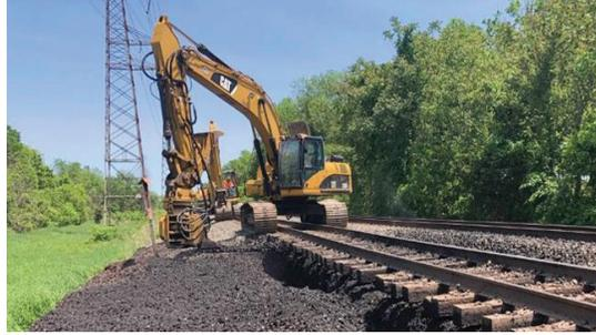
Drainage is one of the most important aspects of track infrastructure. It's important to maintain adequate drainage with proper track ballast to ensure proper cross level, surface and alignment of track. This allows the track to support the loads imposed by rolling equipment.
