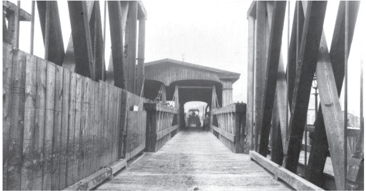
Circa 1898 view of the draw span on the Newkirk Viaduct, which allowed for the navigation of the Schuylkill River. Source: PhillyHistory.org
