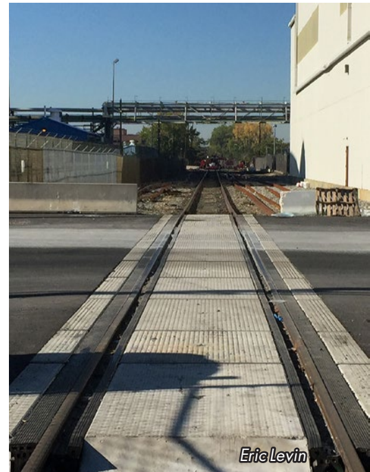
The new Castor Avenue crossing, looking south
